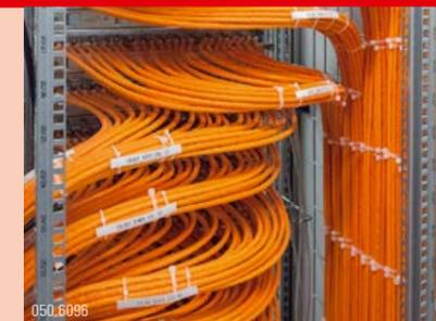
Olten operations control center with computer rooms, 180 server cabinets, distributors and connecting lines features a redundant design. Backbone and access layer of the data network are based on FO cabling. Copper cabling connects the computer rooms with the frontend devices in the control room. Telecommunication is integrated in the Ethernet/IP network.
